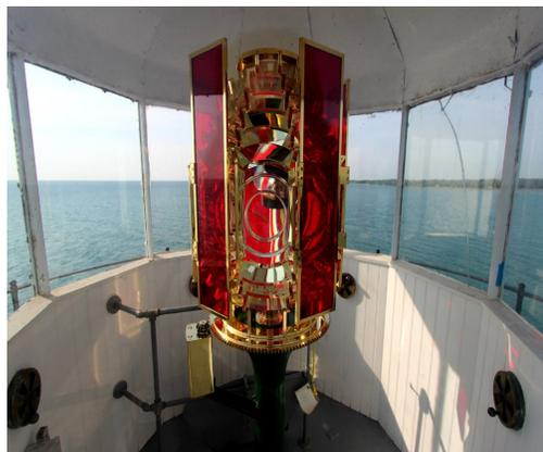
❖ This beautiful 4<sup>th</sup> order Fresnel lens was constructed with prisms made of acrylic instead of glass and is installed in the tower of Harbor Beach Lighthouse in Michigan in 2015 at the cost of \$60,000.
